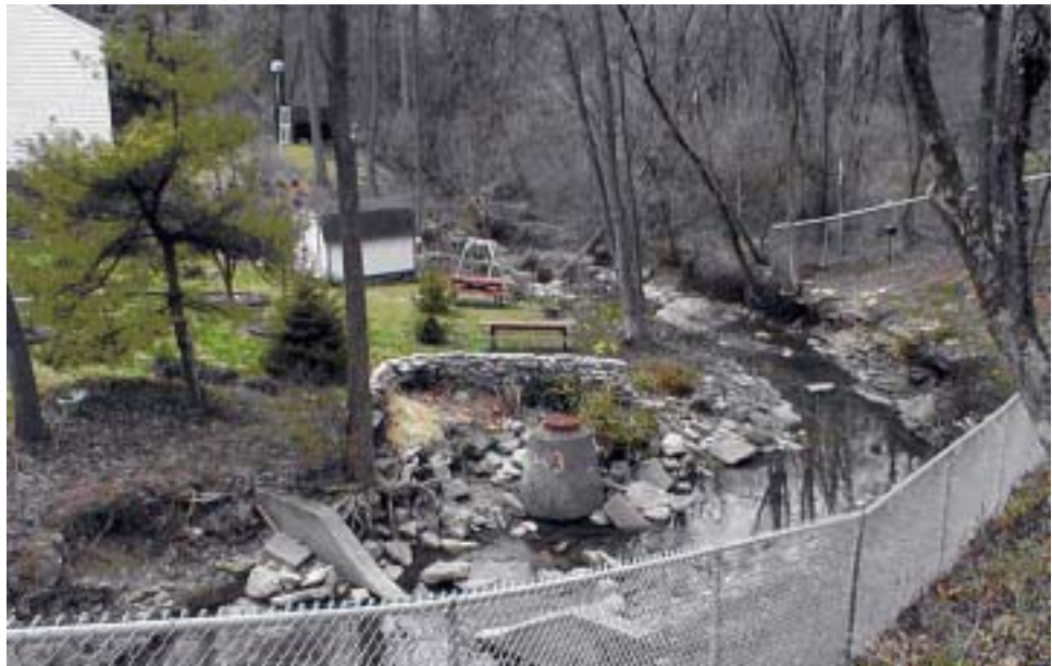
Figure 5 SSO 603 from which raw sewage spilled seven times in 2000 and nine times in 2001 into the E.B. Mill Creek, which flows through residential yards in Hamilton County, OH. 194
