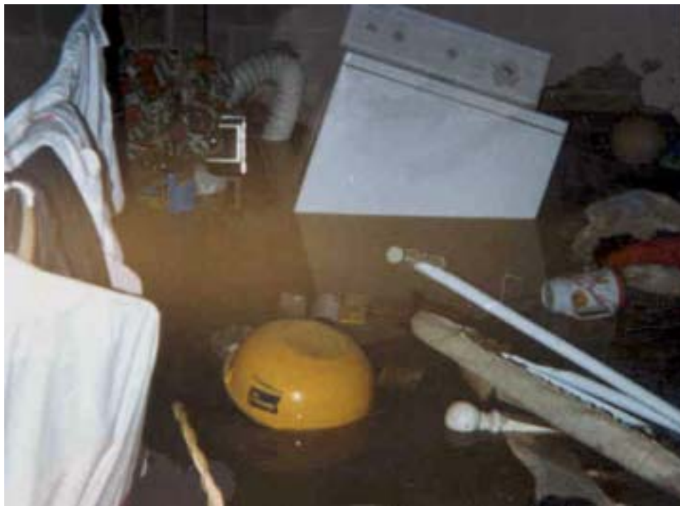
Figure 4 Basement Backup, Cincinnati, OH
