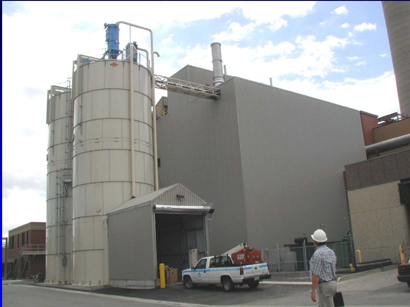
View of the facility (includes finished product storage silos).
