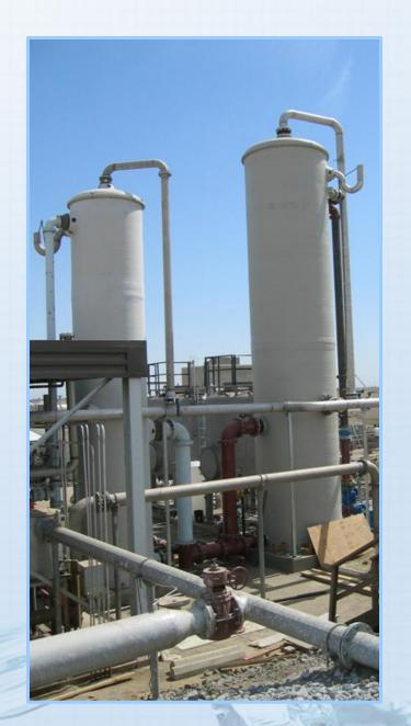
Biogas Biological Trickling Filter Treatment
