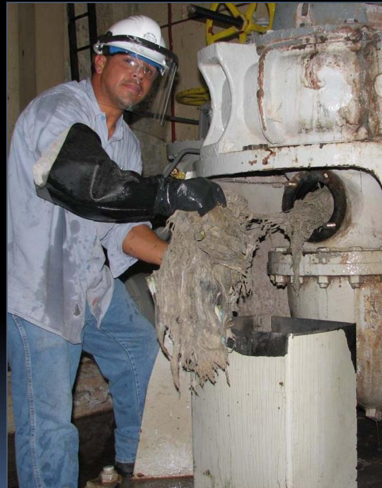
Courtesy Orange County (CA) Sanitary Sewer District
