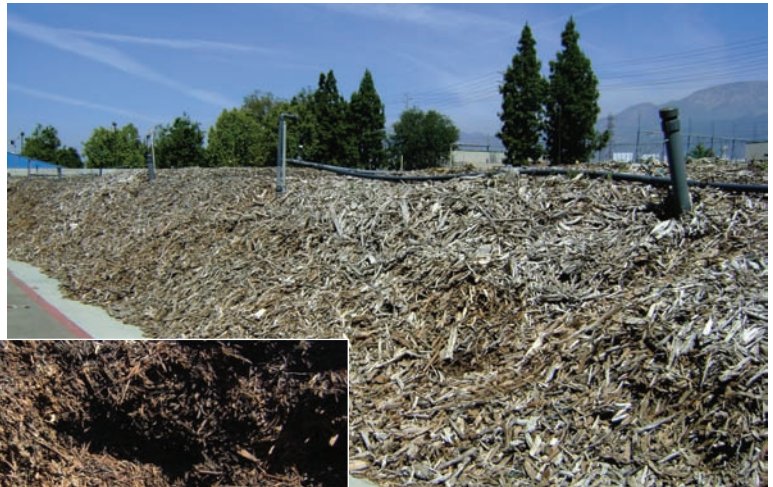
The biofilter contains over 50,000 cubic yards of chipped wood piled onto a perforated floor (inset). Designed air flow rate is 813,200 cubic feet/minute.
