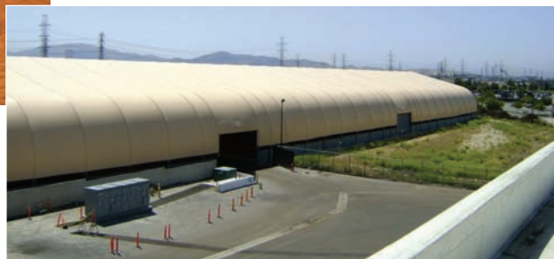
A fabric-covered building can hold nearly three months' production of compost (about 50,000 cubic yards). Storage space is often required during winter months, when sales are slower.
