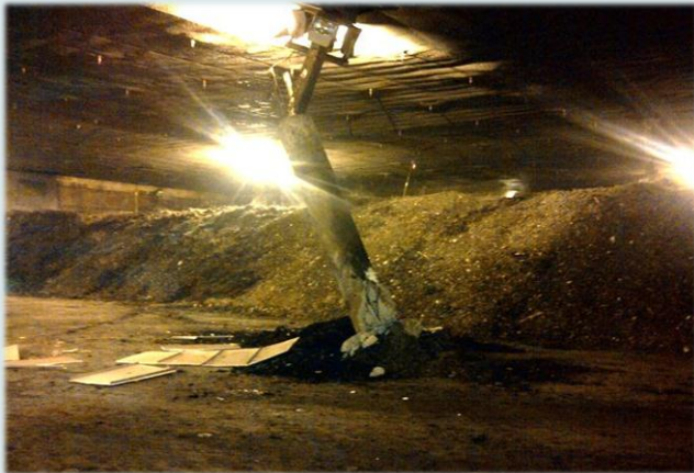
Damaged column, 7/21/2011
