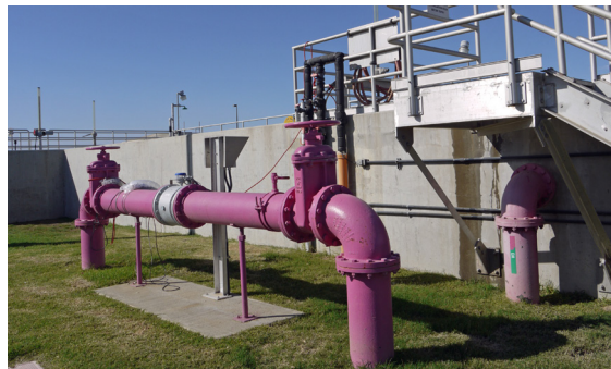
Recycled Water Distribution System
