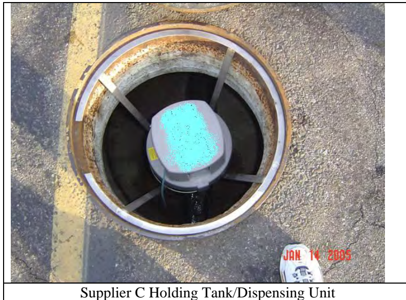
Figure 2.17 Additive Dispenser Setup at OCSD HS27
