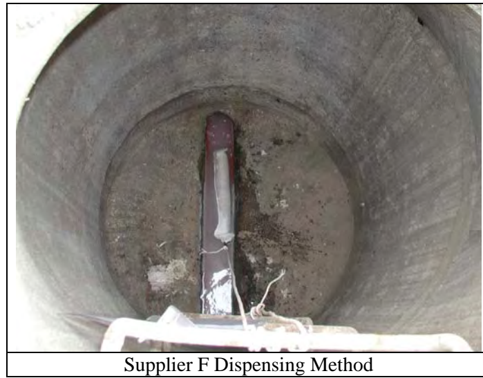
Figure 2.35 Additive Dispenser Setup at COO HS28
