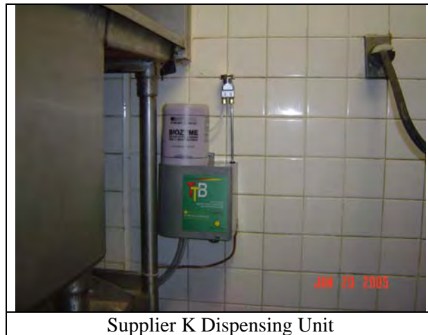
Figure 2.62 Additive Dispenser Setup at CMSD HS14
