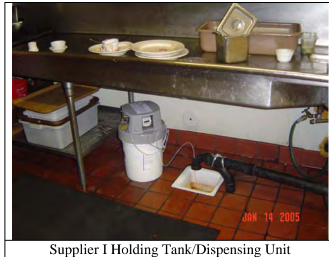
Figure 2.51 Additive Dispenser Setup at GGSD HS106
