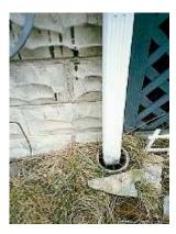
This illegal storm drain connection is an example of a private source of rainwater entering the sanitary sewer system.
