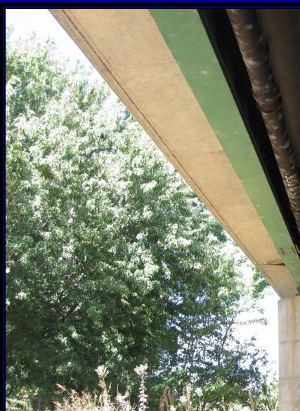
Example: sewer force main crossing over Sacramento River, mounted on highway bridge that previously failed and caused a significant SSO.
