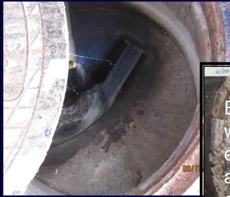
Example: inspection of wet well revealed evidence of substantial accumulation of grease and solids
