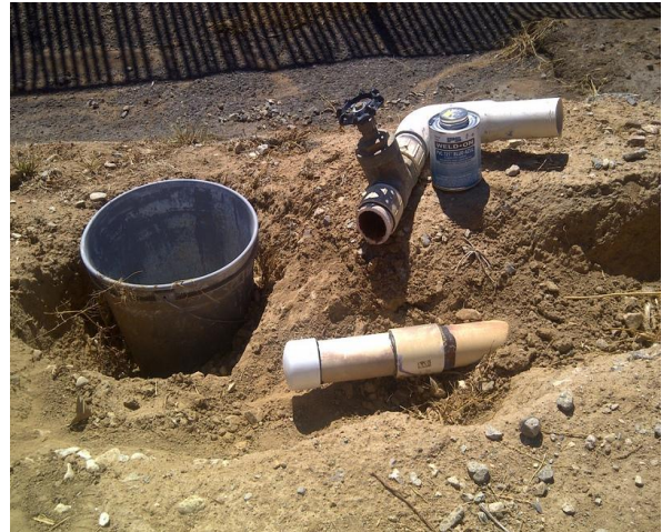
capped drain pipe
