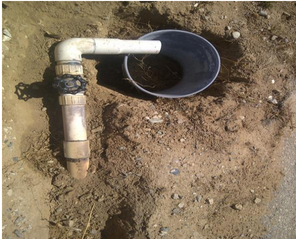
drain pipe emptying into bucket
