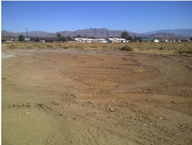
south side of WWTP looking east
